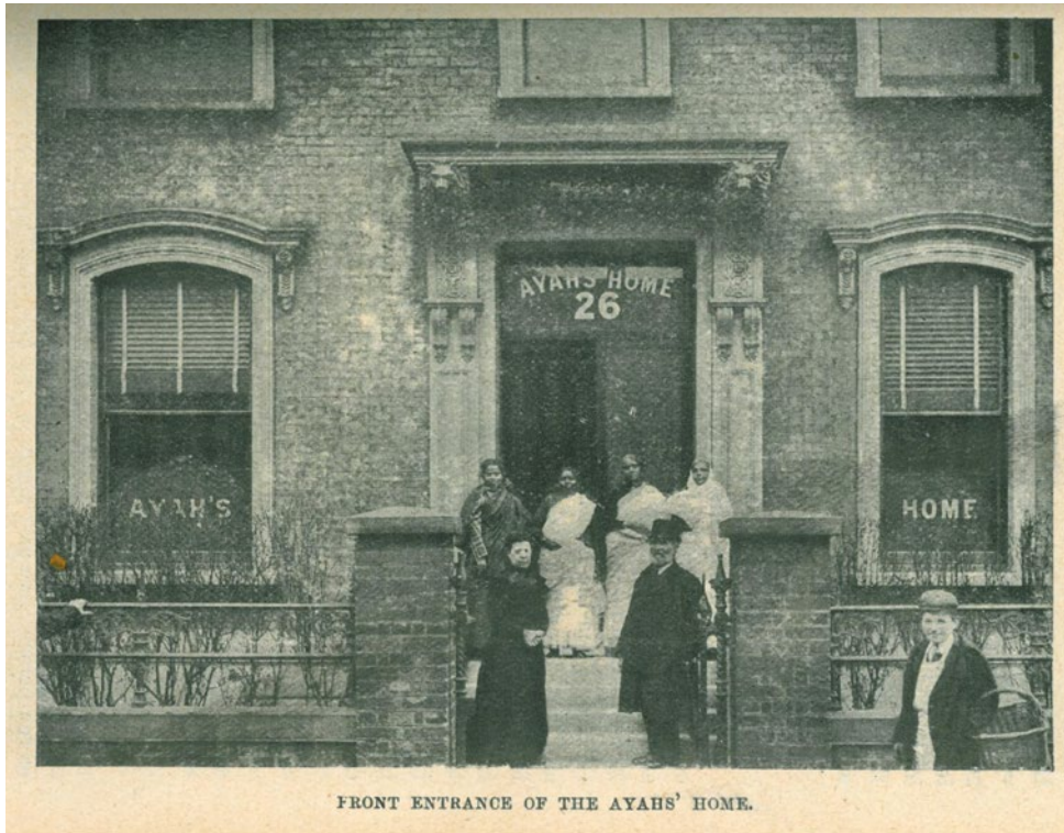
Fig 1 Photograph of the exterior of the Ayahs' Home in Hackney, London City Mission Magazine December 1921 © British Library Board. General Reference Collection PP.1041.C.
